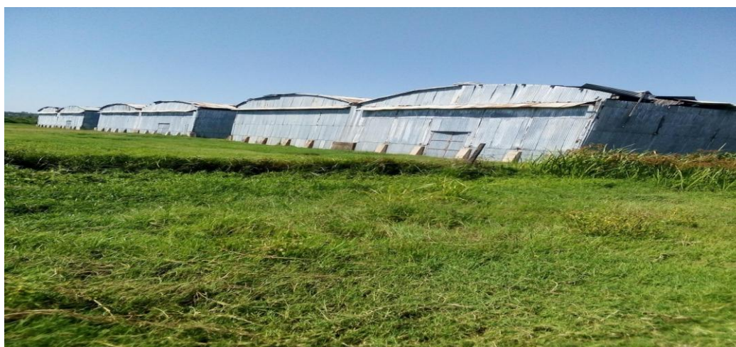
Plate 3.1: Grain Storage Go downs at Kendu Bay (1937)
