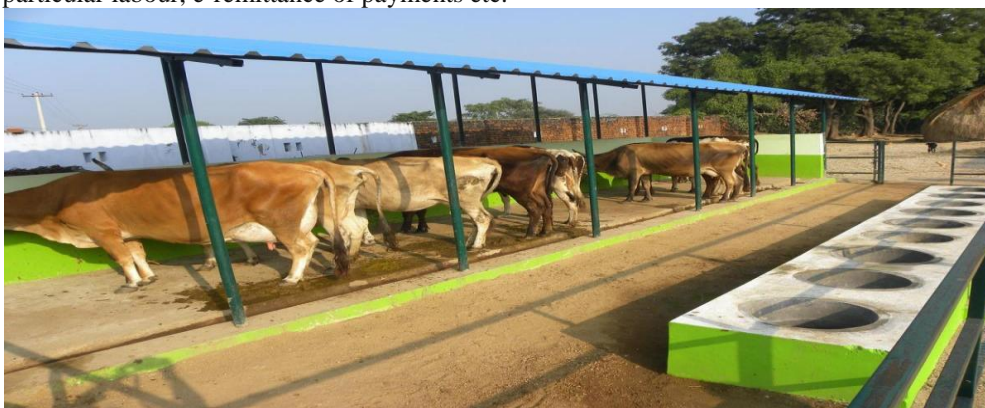
Construction of cattle-shed under MGNREGA in Kolar
