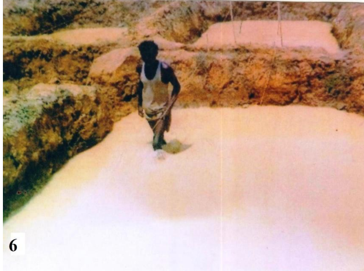
Fig 6: Mixing of special soil in bundh.
